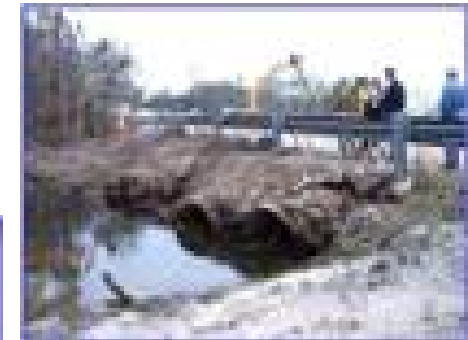
Hurlburt Projects Repairing Hurricane Damage
